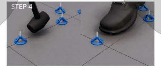
After fixating, wait until the adhesive is dry (24 hours). Then the part that remains on the surface of the coating material should be removed by hitting to the sides of the wedge with screws using a mallet with plastic end.
