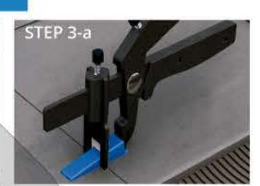
After the coating material is After placing coating material to With the aid of the installation placed on the adhesive, the the empty part of the holder holder joint should be placed joint, wedges should be placed so that it is against the coating to the empty holes of the not exceed the breaking points material and its sole 1 touches holder joint.
